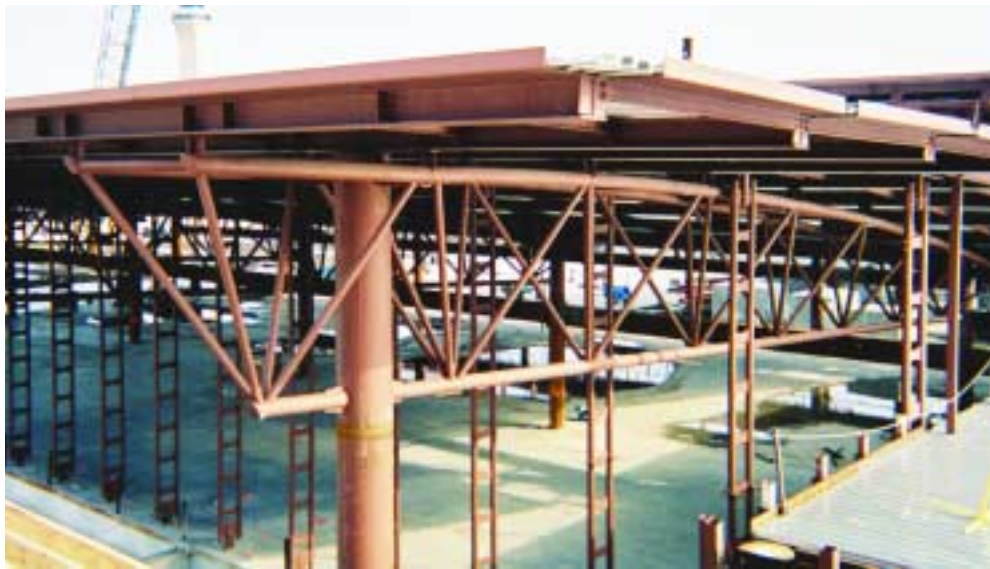
Above: Details of the HSS connections for the tri-chord trusses in the INS Hall. (Details courtesy Walter P. Moore.)
