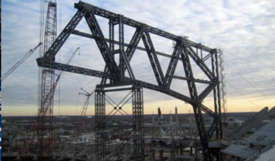
Arched transverse trusses span to two superframes that in turn span parallel to the field sidelines, supporting the entire roof without compromising sightlines.
